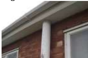
Fig 3 Asbestos Cement drainage pipe
