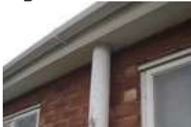
Fig 3 Asbestos Cement drainage pipe
