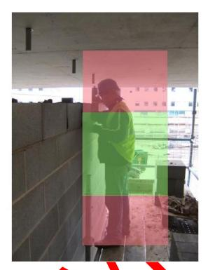
Arrange working platforms so that block laying can take place between chest and knee height. In the illustration above the green zone represents the area in which a worker can lay blocks with a maximum weight of 20kg at a typical rate of up to 20-30 units an hour.
